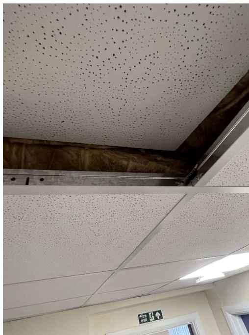
Photograph Four – Roof Insulation
